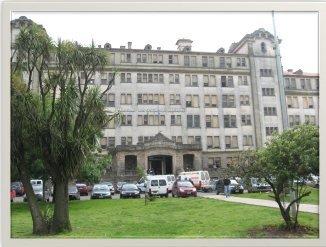
HOSPITAL INTERZONAL GENERAL DE AGUDOS
